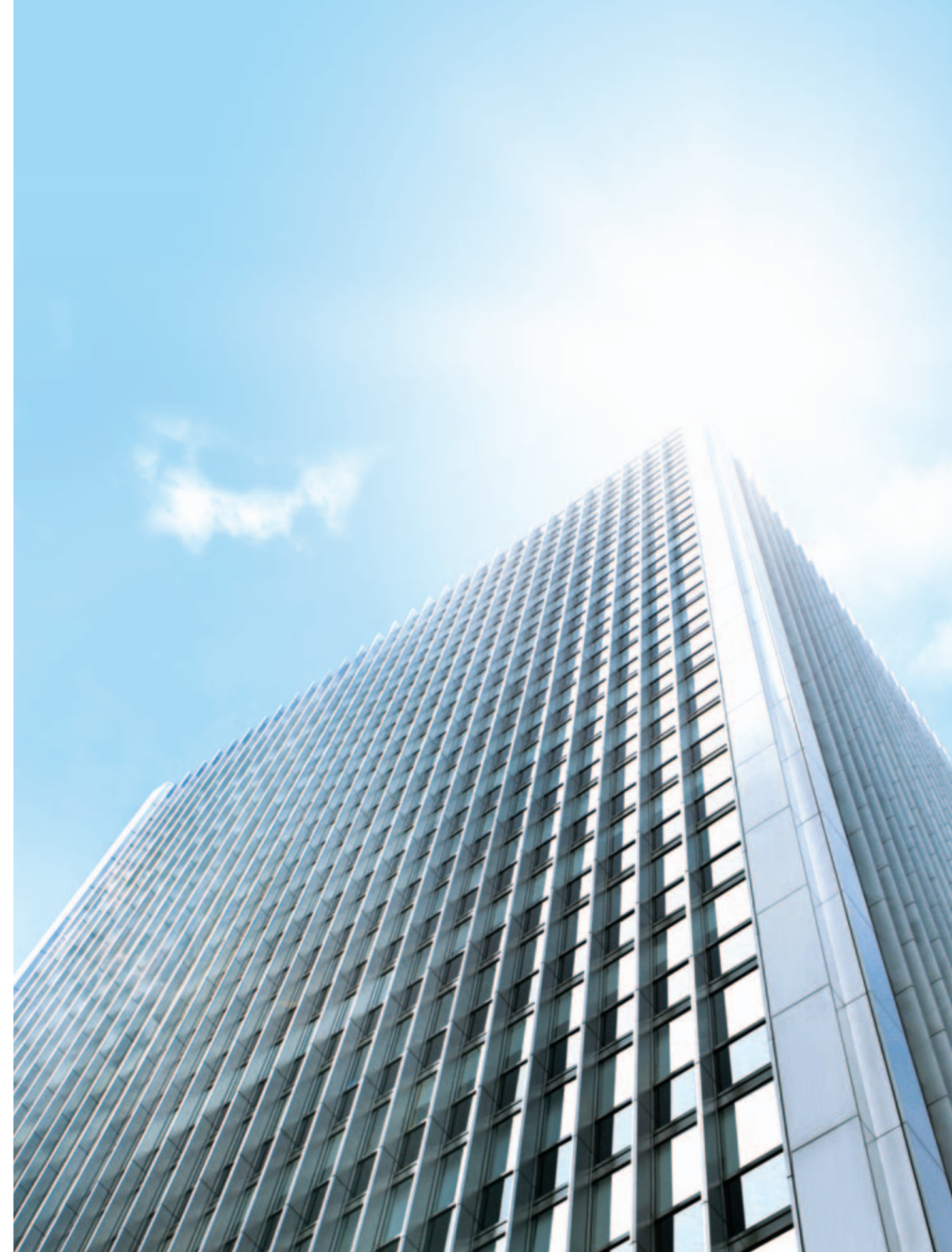
Wheelock House Pedder Street, Hong Kong
